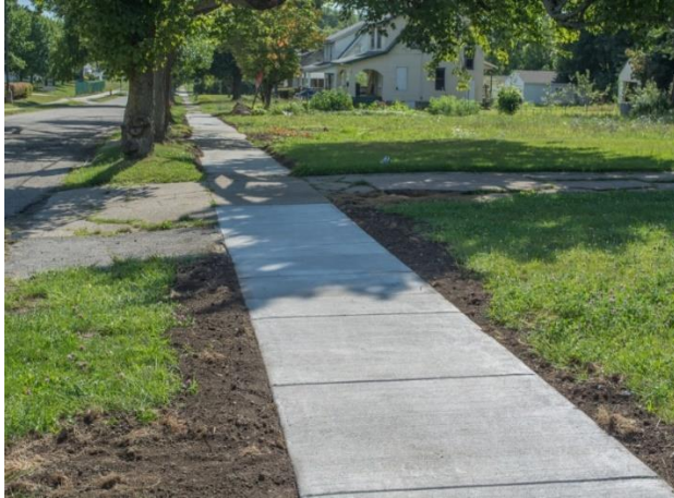
Sidewalks were installed around Taft Elementary School as part of the Safe Routes to School Program in 2017, connecting the school with sidewalks leading to nearby Homestead Park
